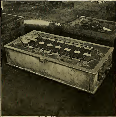
Fig. 62. Drag Half of Mould with Cores Set.
